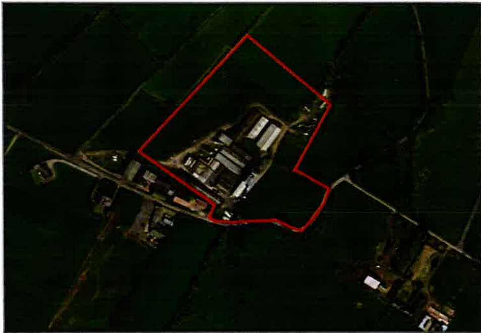
Figure 4 – Aerial Photograph of the Site (Outlined in Red) and its Surrounding Habitats © Google
